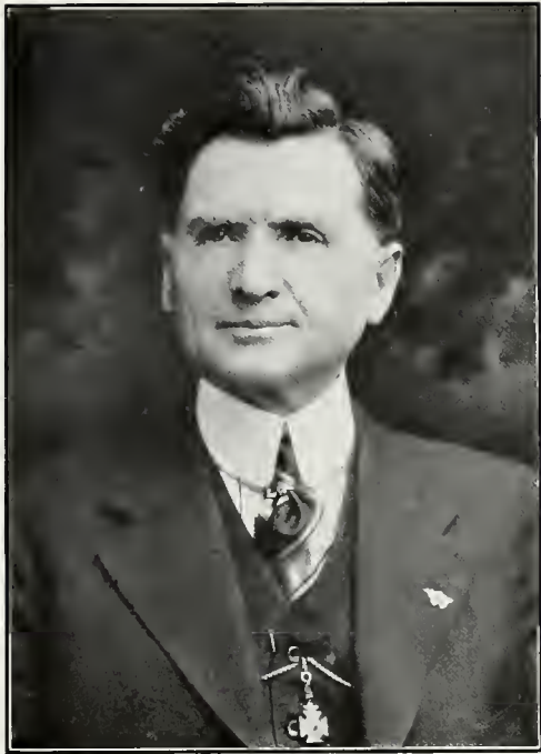
MARSHALL RUST CONTRACTOR
